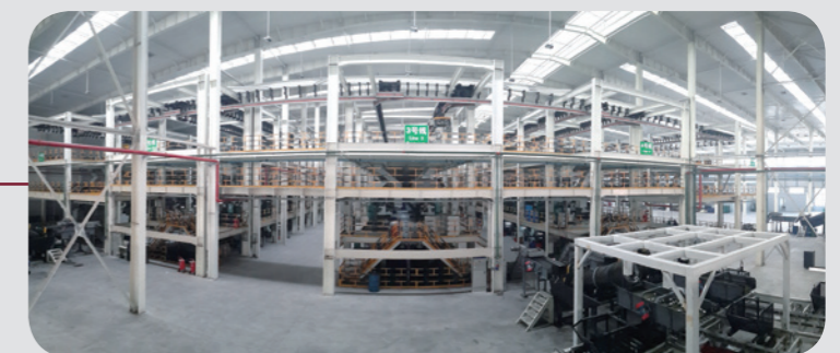
Threading, Air Pressure Test, and Anti-rust Treatment
